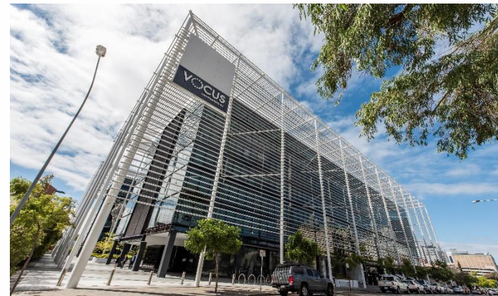
Workzone West, Perth, WA
